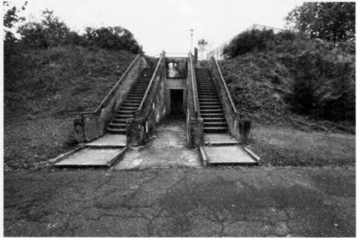
One of two emergency exits from the bunker
